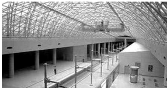
Figure 17: View of the station at Incheon International Airport (Source: www.en.wikipedia.org . Incheon Airport)
