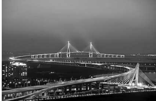
Figure 14: The 7-mile long Incheon Grand Bridge between Songdo and the Airport (Source: www.songdo.com )
