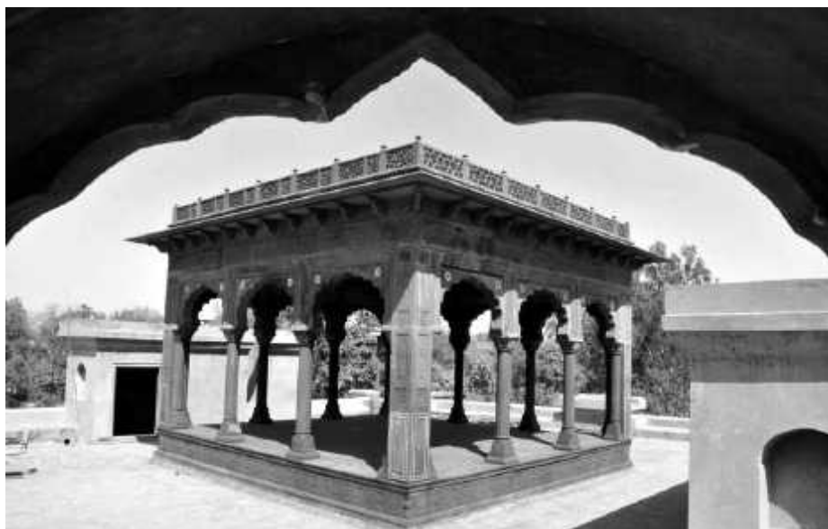
Figure 11: The Baradari after completion of conservation. (Source: ASI)
