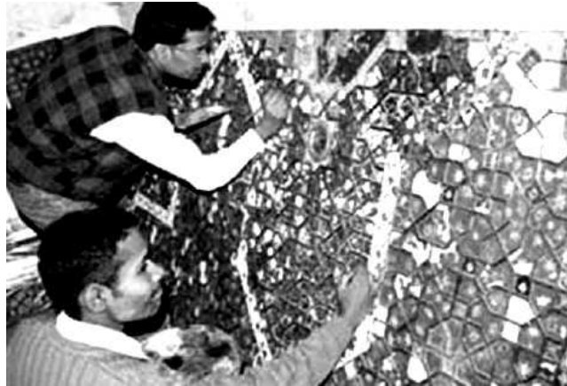
Figure 9: Restoring the Khatamband ceiling
