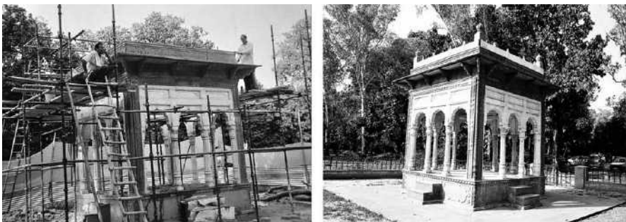
Figure 18: Chhoti Baradari, during and after reconstruction
