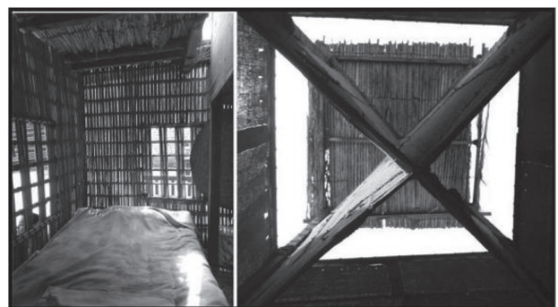
Figure 4: Interiors of tradition vernacular homes of Dubai (left), Windcatcher (right) (Source: Author).
