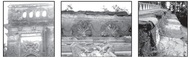
Figure 30: Growth of several strangler figs in the building. (Source: Photographs taken by the authors).
