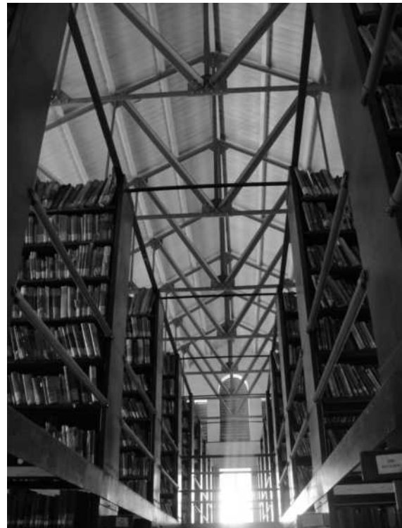
Figure 10. Stacks and truss systems (Image Source: Author, 2011).
