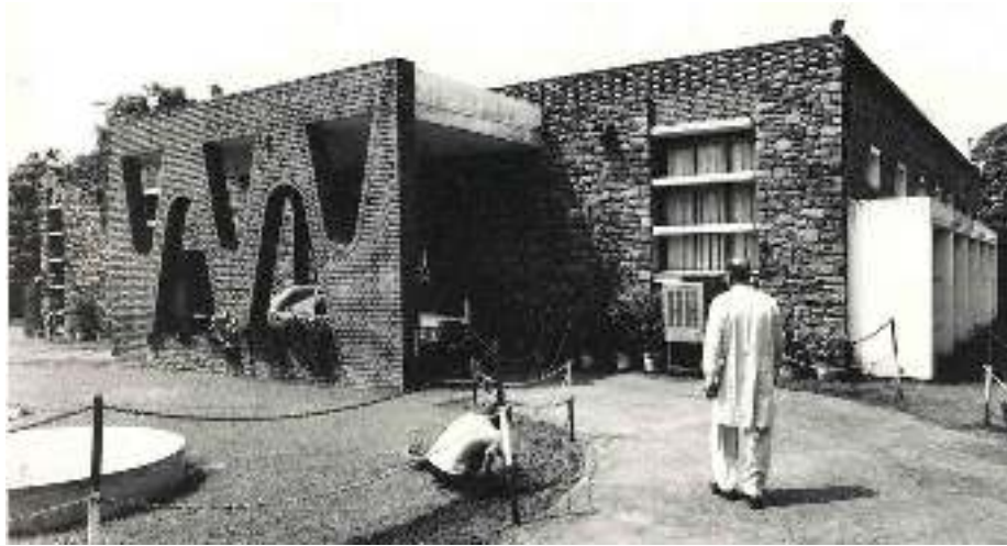
Figure 1 (Previous page): Some of the smallest houses designed by Pierre Jeanneret. Projecting bricks animated the simple facades while shadows cast by the projections helped to lower temperatures.
