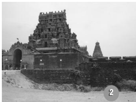
Figure 5: Thanjavur Viewpoint V2 -- Immediate view of Vimanam from the north-eastern side -- Big Temple Road (Image Source: P. Gopalakrishnan)
