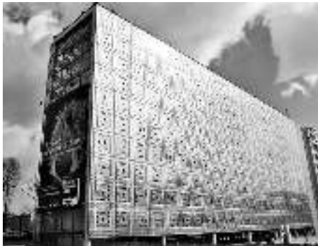
Figure 5a and 5b (Above Left and Right): KfW Westarkade in Frankfurt, Germany designed by Sauerbruch Hutton (Image Source: - http://www.archello.com/ )
