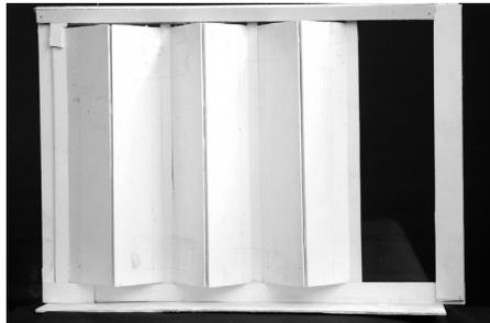
**Figure 5 (Top):** Model of a 'Timber Sliding-folding Door,' made to understand the mechanism involved
