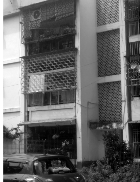
Figure 4: Use of concrete jali in staircases does not prevent access of lashing rain but reduces light and ventilation in stair halls.
