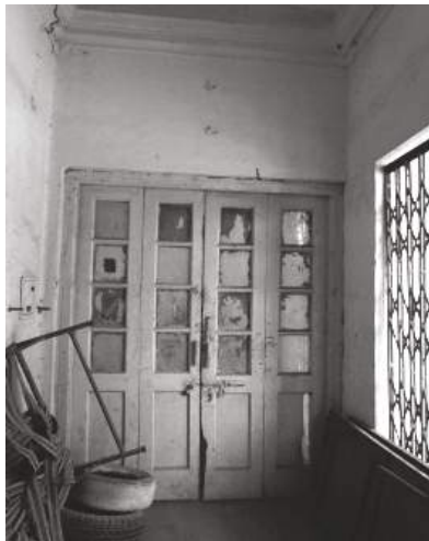
Figure 31. Wooden door, with glass and wooden panel infill (Source: Clicked by Author).
