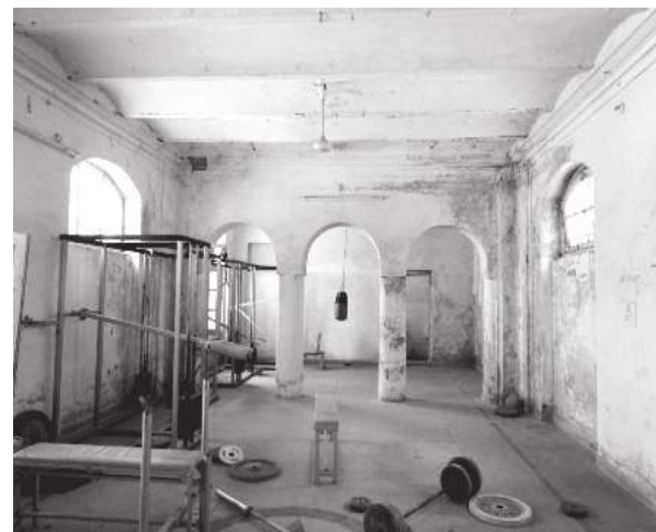
Figure 28. Kota stone as a flooring material, which is laid later on. Huge thick circular columns inside the room to share the load. (Source: Clicked by Author)..
