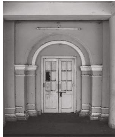
Figure 33. Wooden entrance door, inscribed in double arches which are supported through huge pilasters (Source: Clicked by Author).
