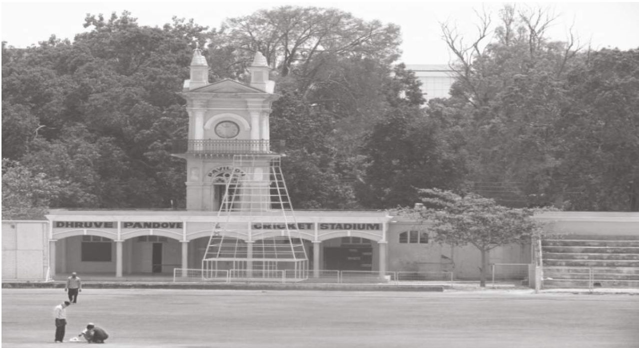
Figure 24. DhruvePandove Pavilion cum Stadium (Source: Clicked by Author).
