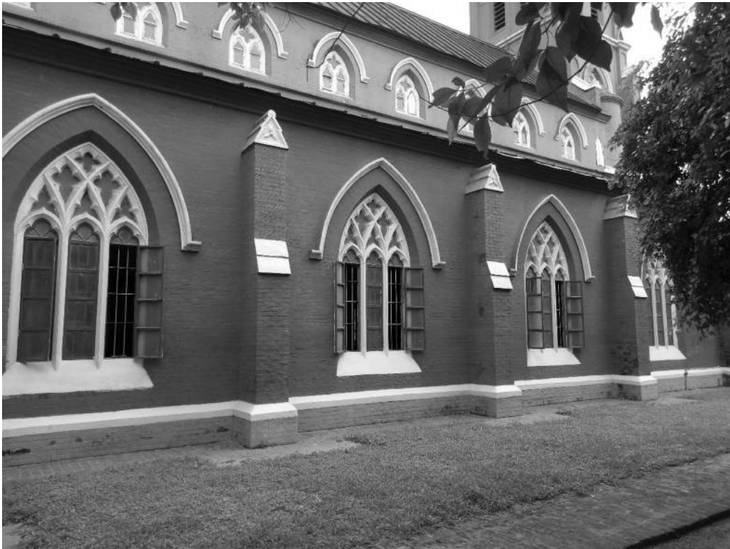
Figure 9. Pointed Gothic windows spread symmetrically on the facades (Source: Author)
