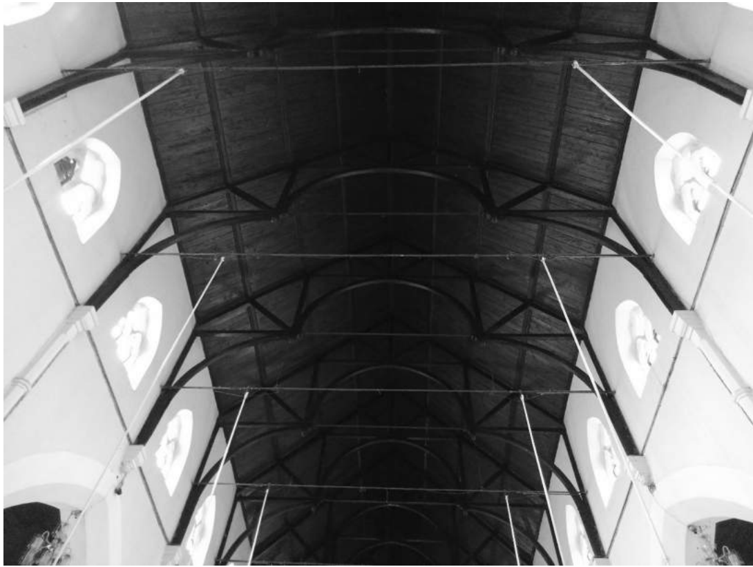
Figure 11. The oofs with wooden trusses and wooden planks (Source: Author)
