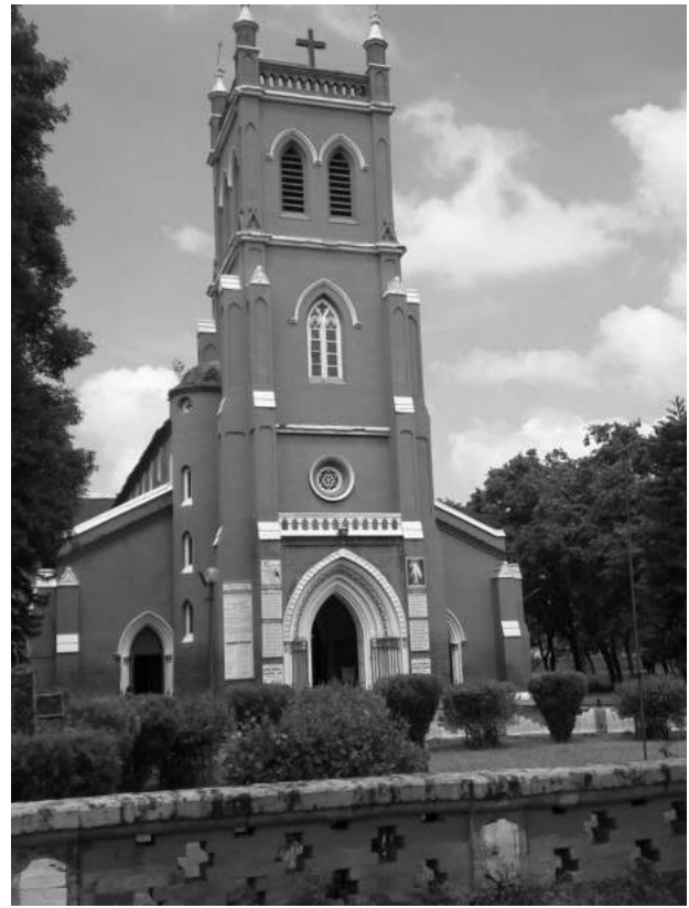
Figure 7. The exterior view of Holy Redeemer Church, Ambala Cantonment (Source: Author)
