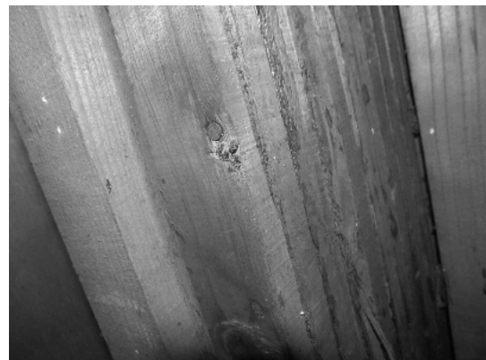
Figure 4. The Plywood Structure for the Public Hall (Source: Author, 2012).
