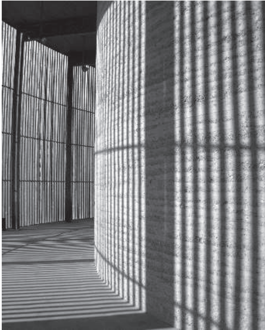
Figure 18: The Chapel of Reconciliation was designed with respect to the physical and historical context by Berlin Architects Reitermann and Sassenroth, and constructed by the local mud-building expert Rauch. The raw state of materials, structural and atmospheric, deeply engages inhabitants. The 30cm thick rammed earth walls visibly comprise local clay and pieces of stone and glass from the rubble of the previous church. The journey inwards is defined by materiality; the inner space between permeable timber vertices and solid earth wall is penetrated by streaks of light and a gentle breeze, creating a sense of reflection. [Source: Photograph by the author]
