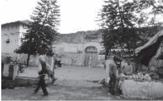
Figure 7: Deteriorating condition of Tehsil office in Hamirpur town, H.P.
