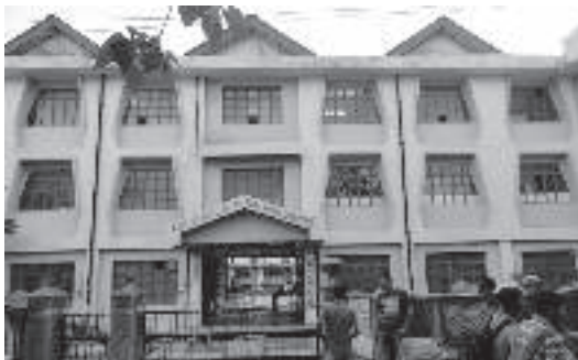
Figure 10: View of the Government Senior Secondary School with good architectural quality
